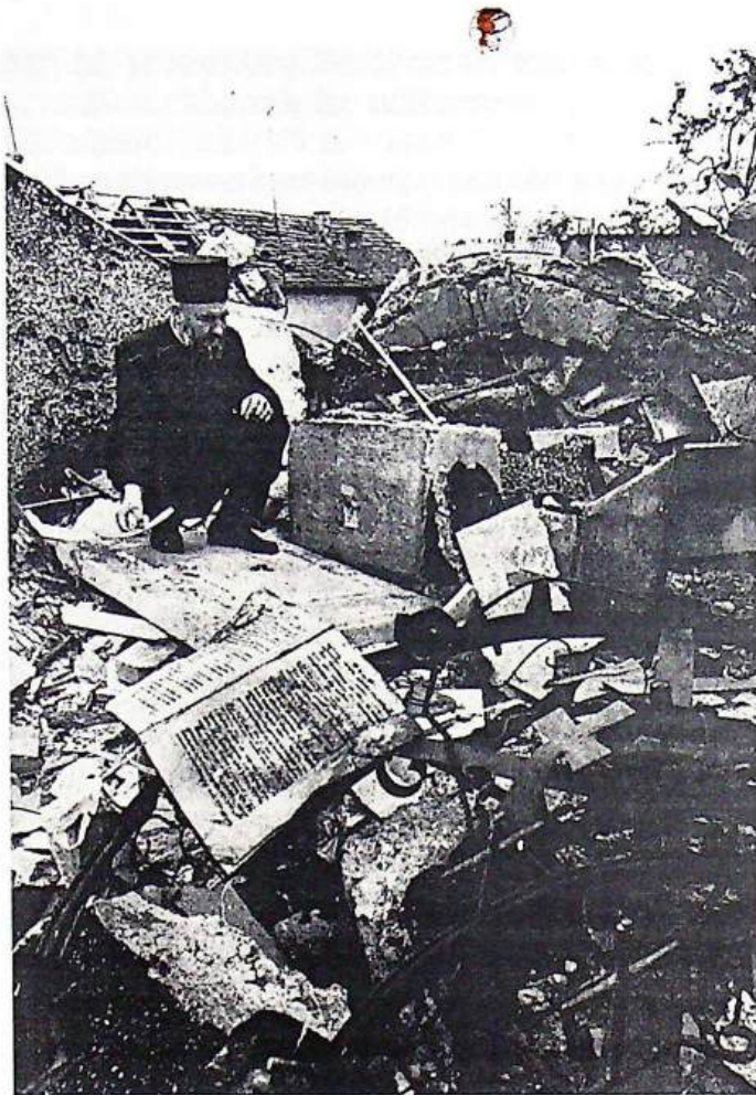
A destroyed Orthodox church in Petrinja.
