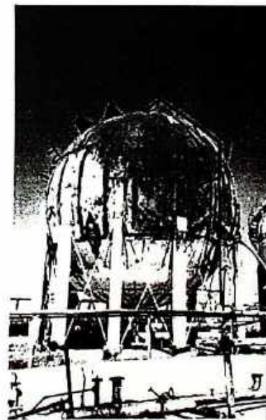
Damaged VCM tank at the petrochemical plant in Pančevo
